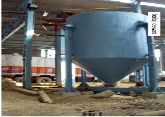
ROCK STORAGE TANK
